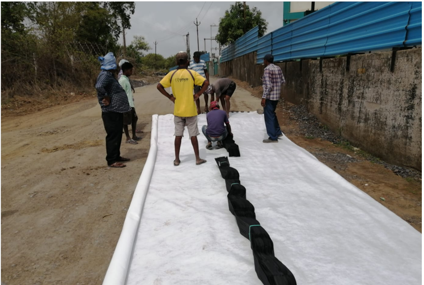
Photo 4 : Placing Techcell Geocell over Nonwoven Geotextile
