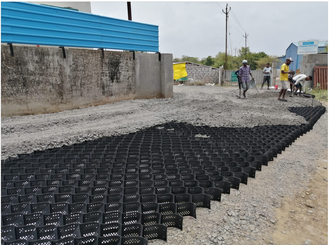
Photo 7 : Filling Geocell with GSB Material
