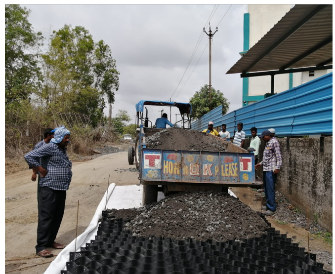
Photo 6 : Filling Geocell with GSB Material
