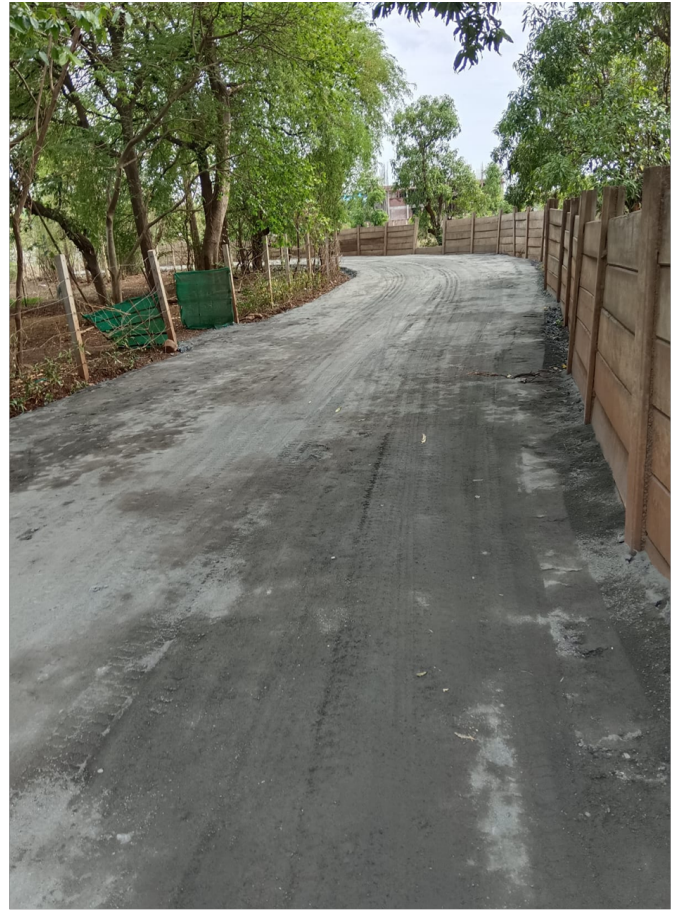
Photo 9 : Finished View of the Road
