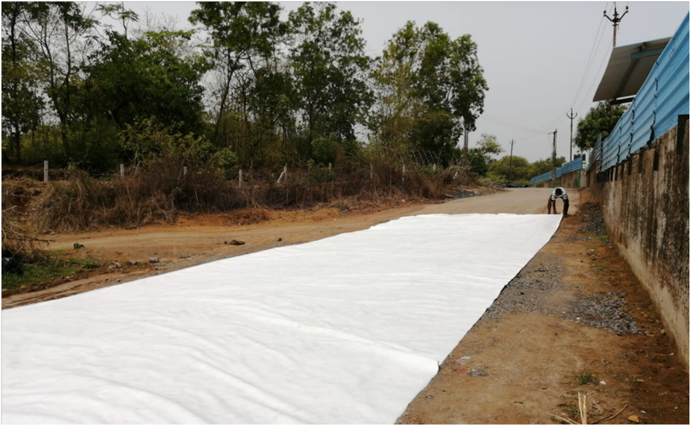
Photo 3 : Laying of Non woven Geotextile as Base Material
