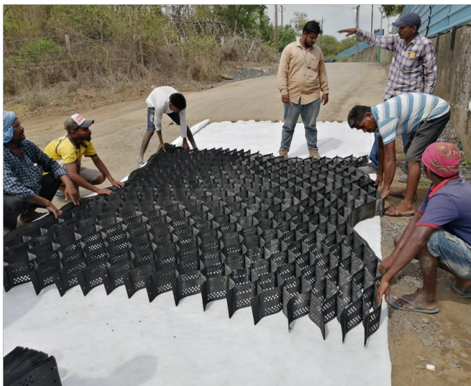
Photo 5 : Expanding & Fixing of Geocell Layers
