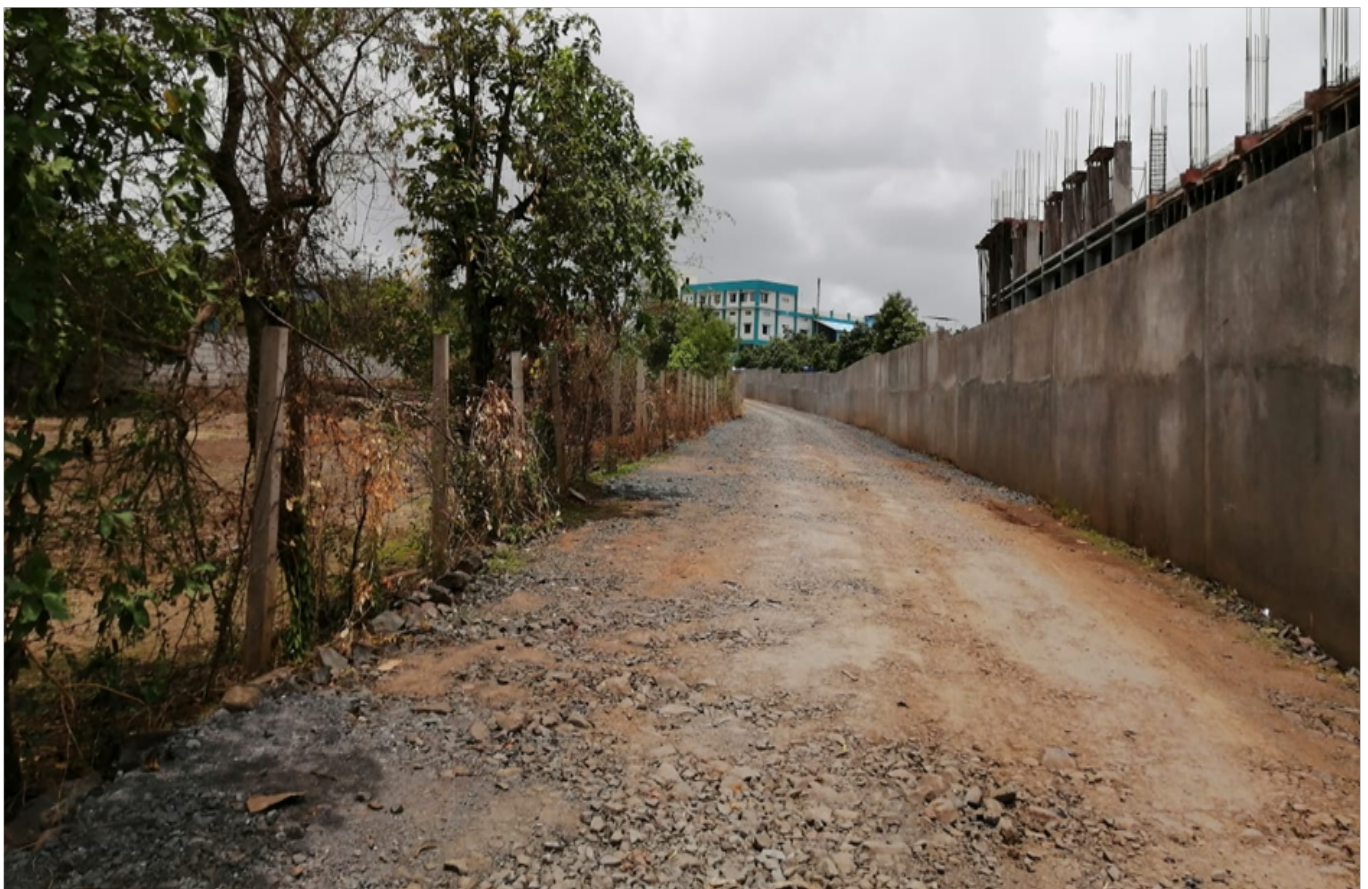
Photo 2 : Laying of GSB and Dressing the Road
