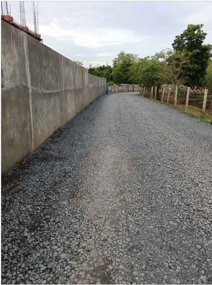
Photo 8 : Road After Rolling & Compaction
