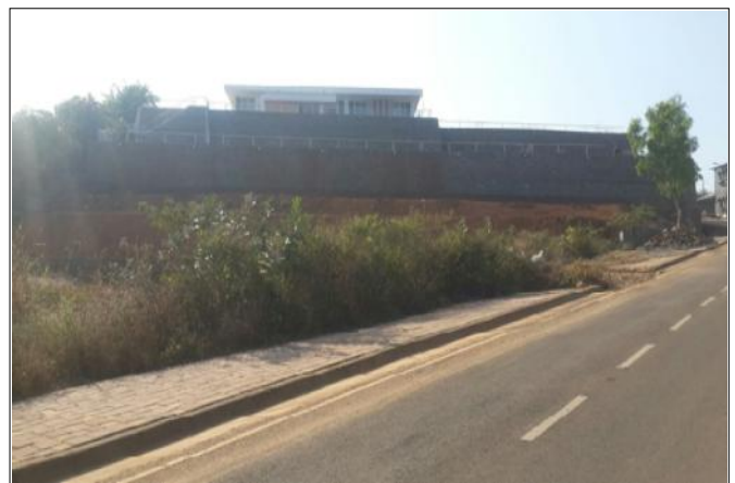
Fig 5 : After Construction - View from far
