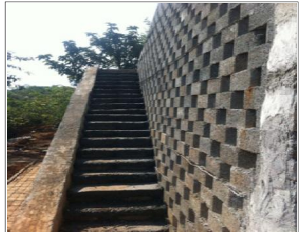
Fig 2 : Stairs over reinforcement
