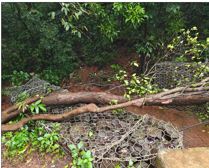
Photo 1 & 2 : View of TechFab Metal Gabion Retaining Wall
