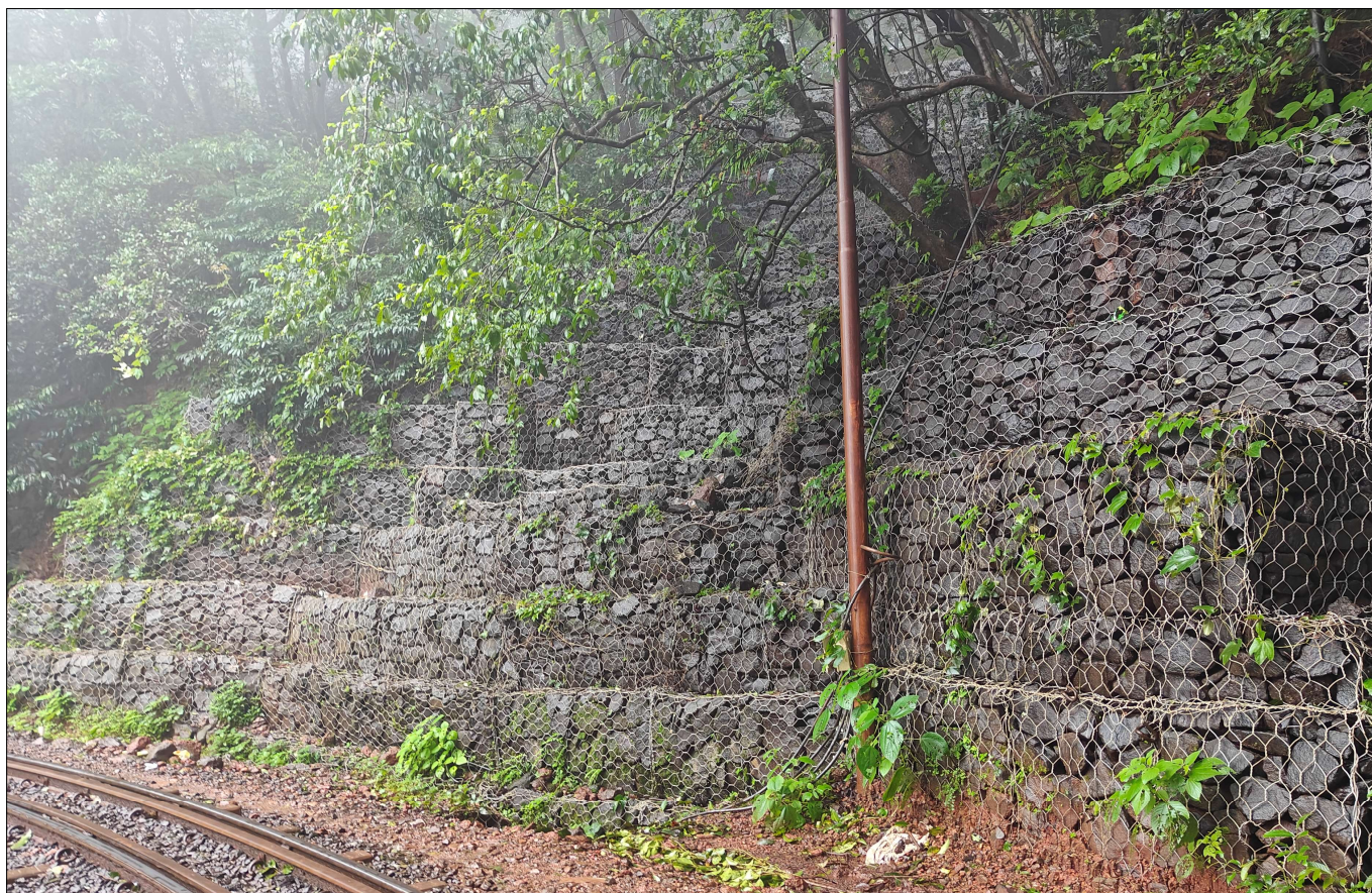
Photo 3 : Gabion Wall for Slope Retention on Hillside
