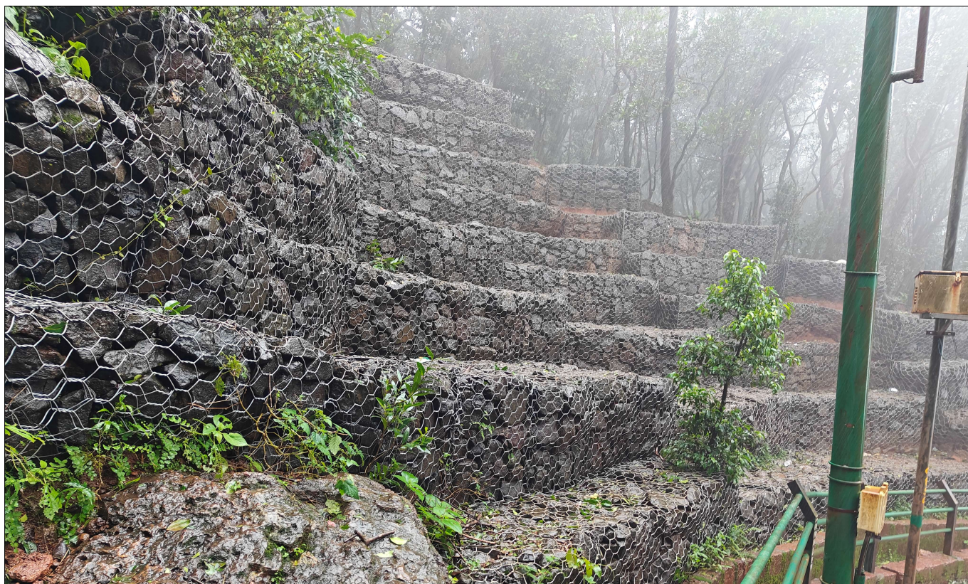
Photo 4 : Eco-Friendly Gabion Wall: Strengthening Hillside Slopes Naturally
