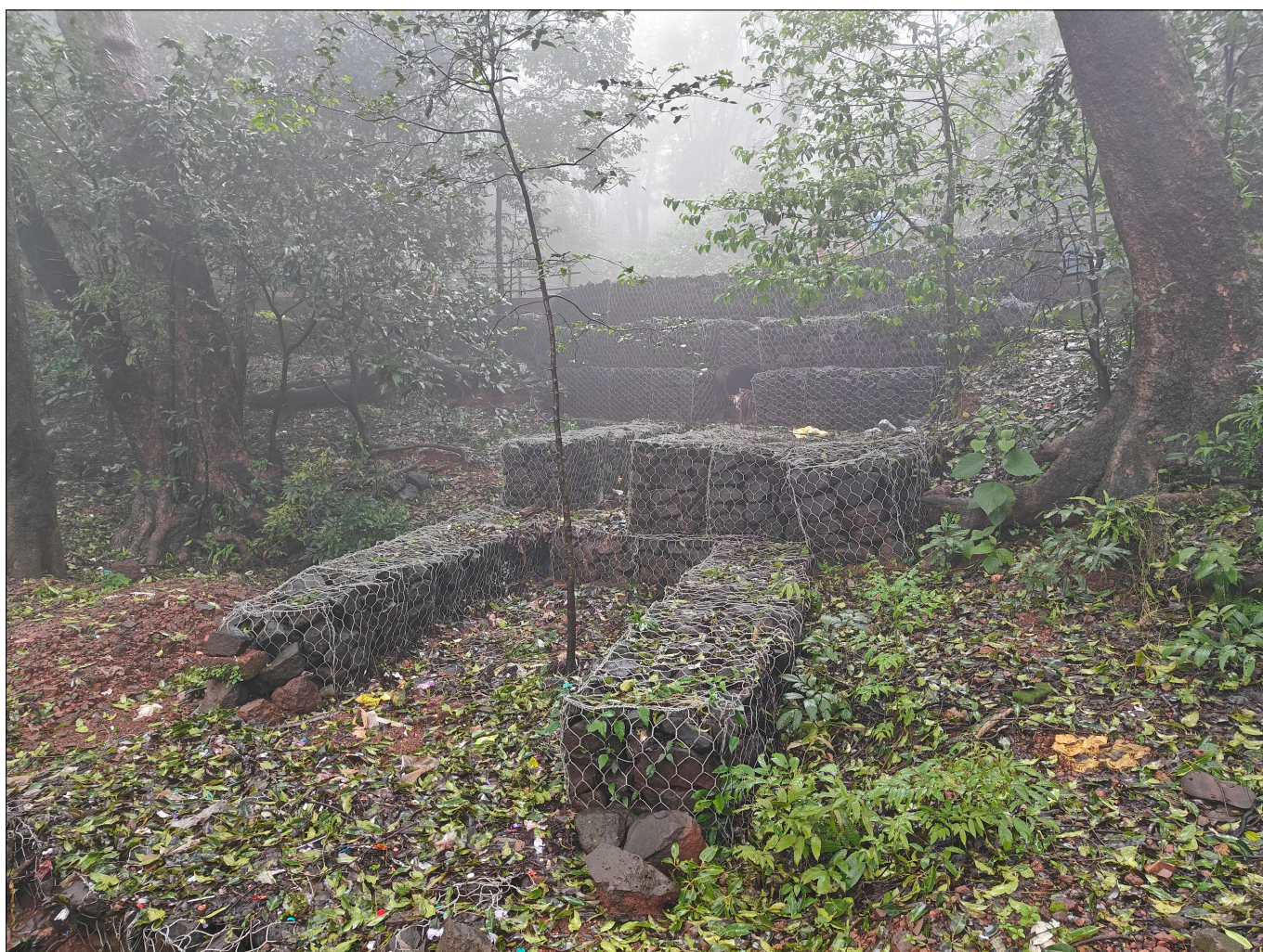
Photo 5 : Enhancing Drainage with Gabion Culvert Solution
