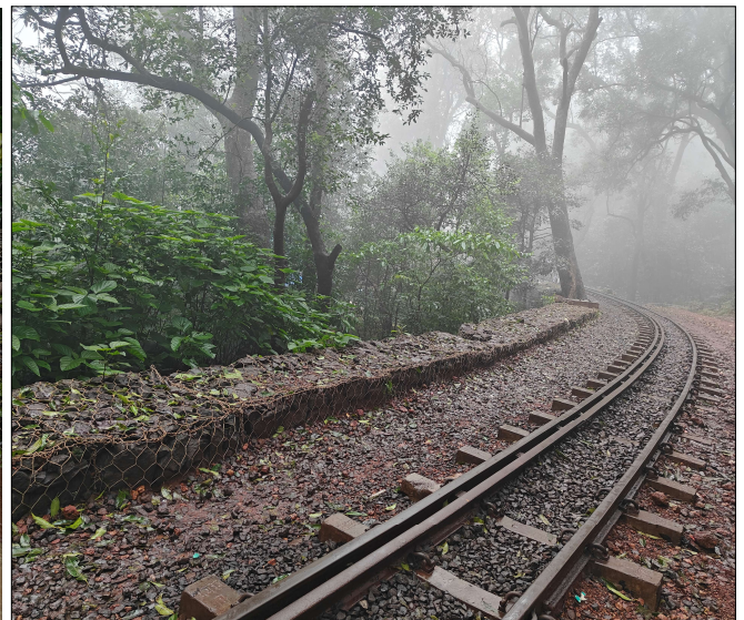
Photo 1 & 2 : View of TechFab Metal Gabion Retaining Wall
