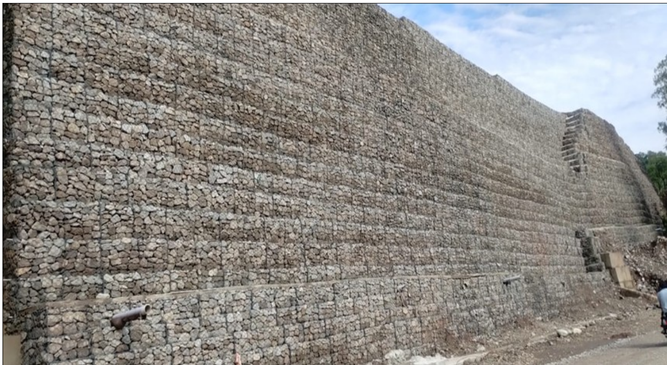
Photo 4 : Completed RS Wall with effective drainage measures
