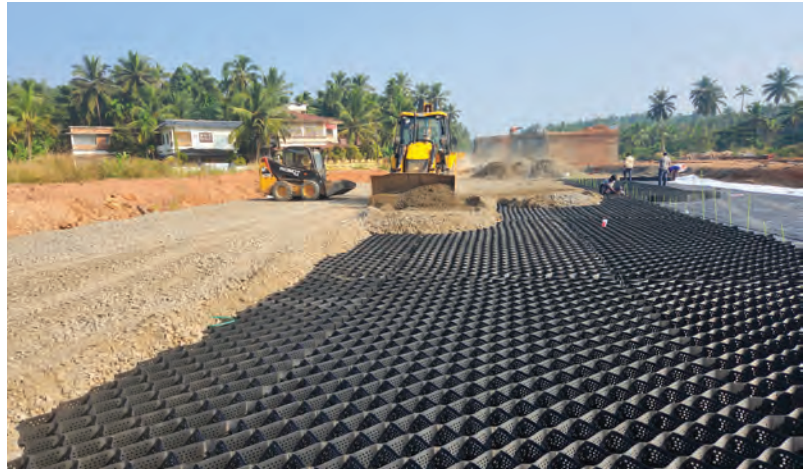
GEOGRID INSTALLATION BENEATH A GRANULAR WORKING PLATFORM
