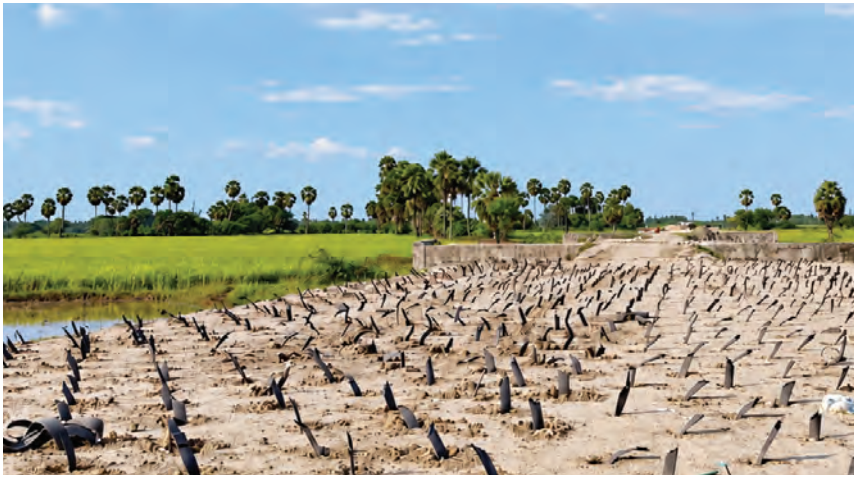
PVD INSTALLATION ACROSS A SOFT GROUND TREATMENT AREA
