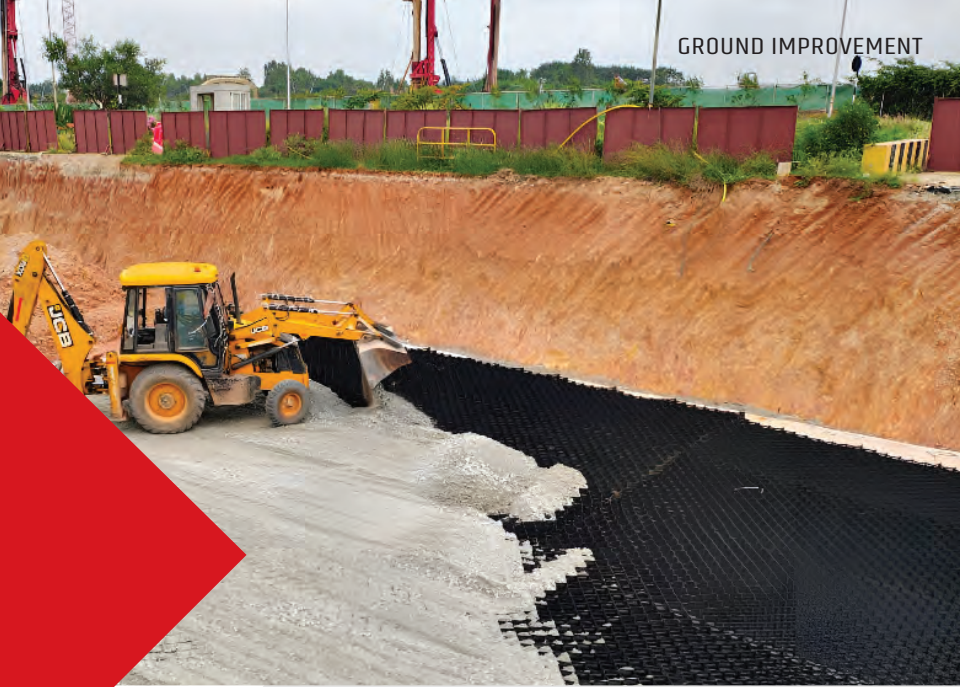
BASAL SEPARATION LAYER PLACEMENT - EMBANKMENT FOUNDATION PREPARATION
