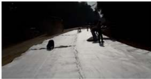
Figure 3: Overlapping of Drainage Composite ends with the adjacent rolls
