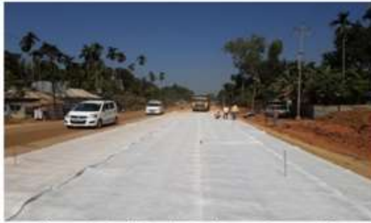
Figure 2: TechDrain Drainage Composite Unrolled on the Stabilized Sub Base
