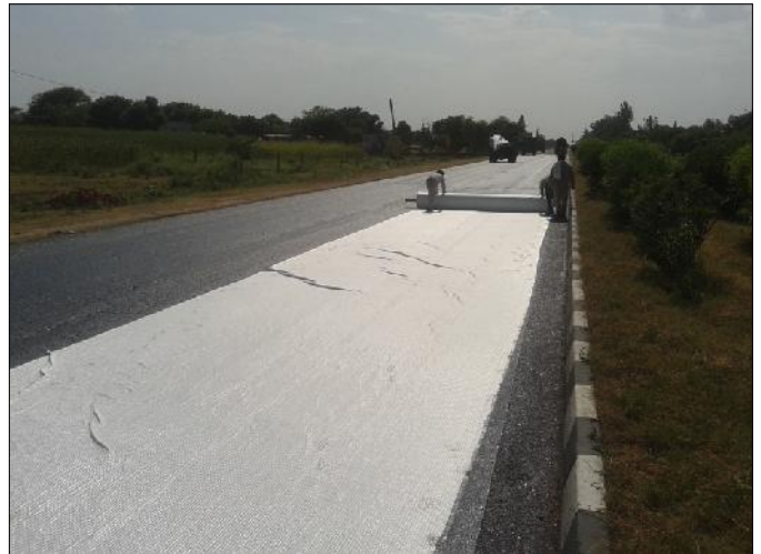
Laying of Geotextile
