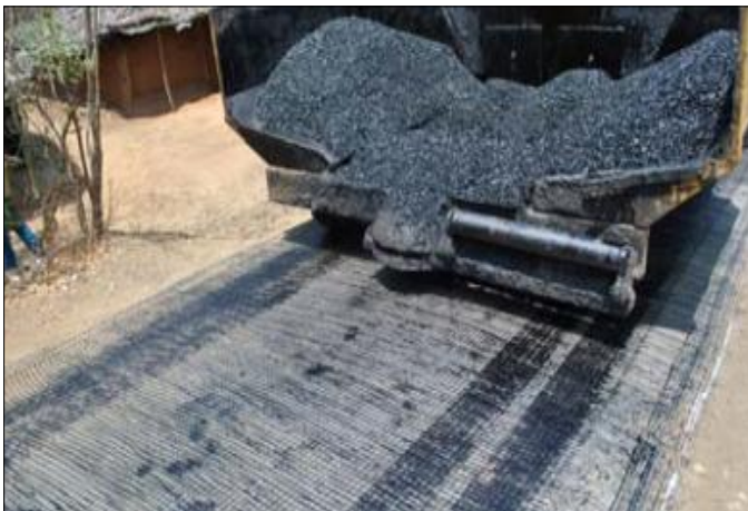
Over lay being laid over the TechGlass
