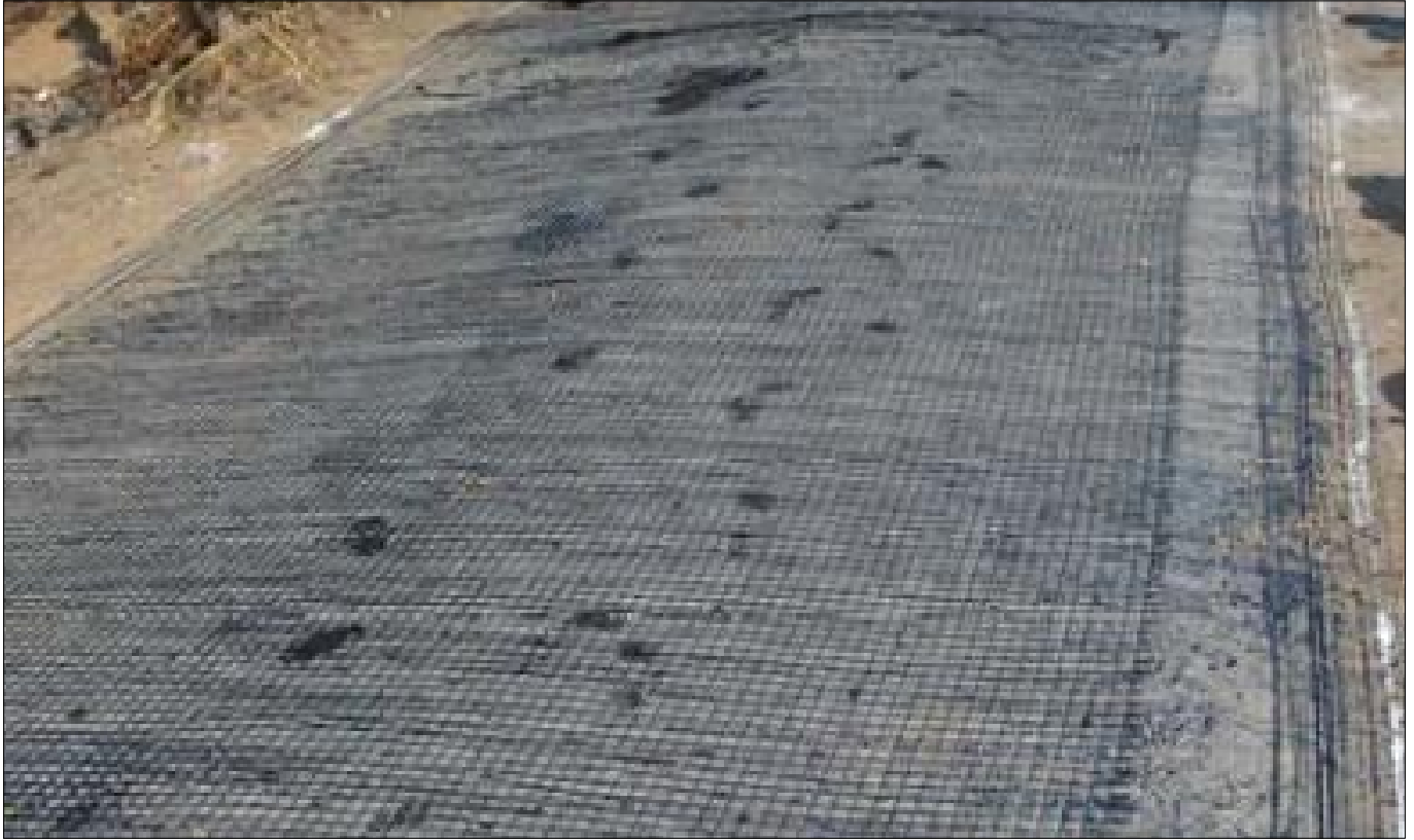
Laying of TechGlass 50
