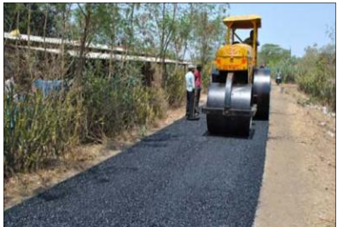
Compaction of Over Lay
