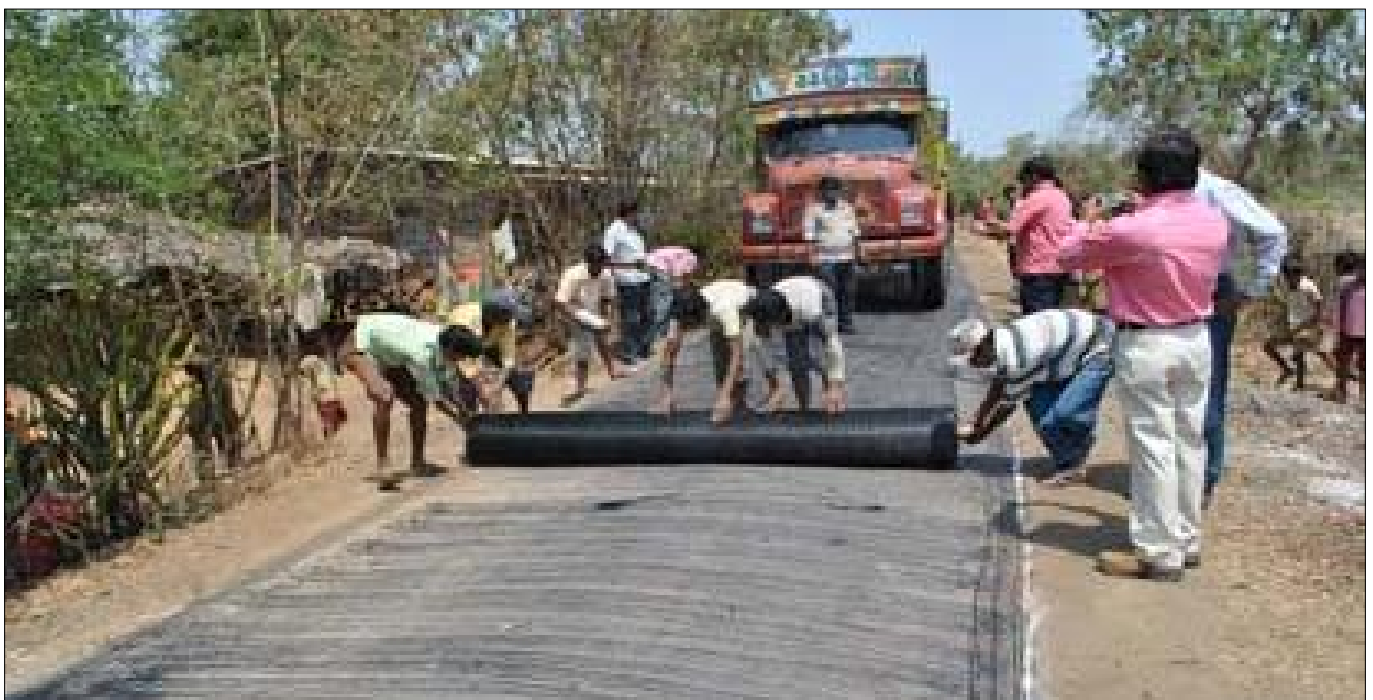
Unrolling of TechGlass 50 at the site
