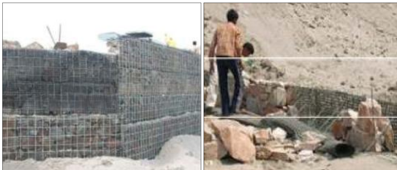
During Construction Photographs
