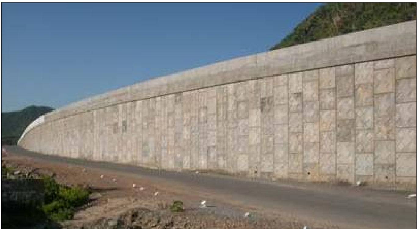
Photo 1 : Elevation view of RS Wall
