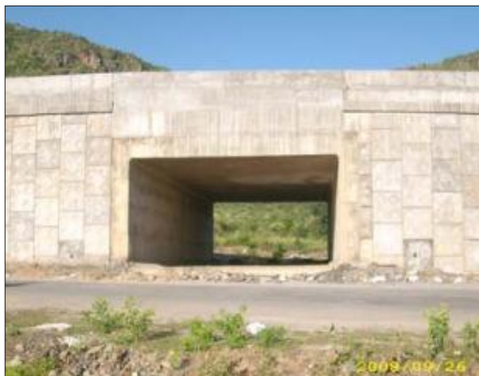
Completed RS Wall
