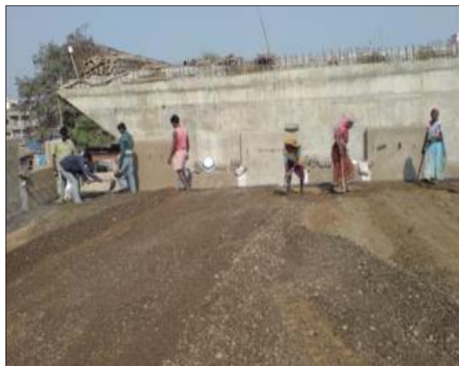
Erection of RS Wall
