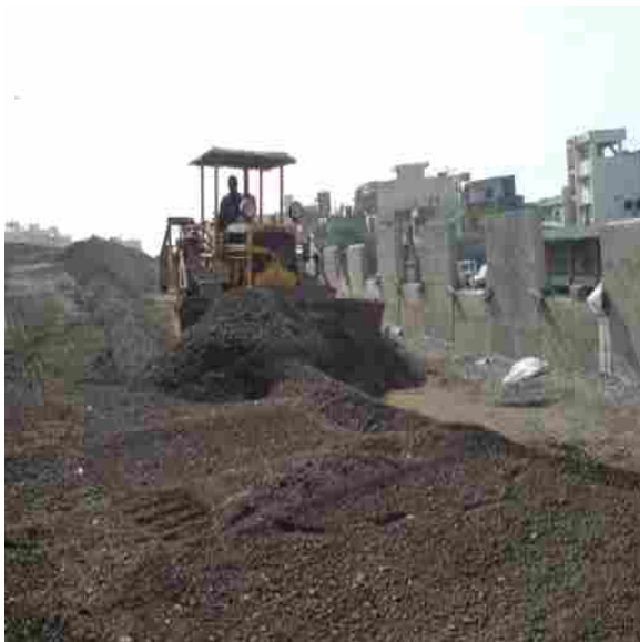
Photo 5. Spreading and Compacting the Reinforced Fill
