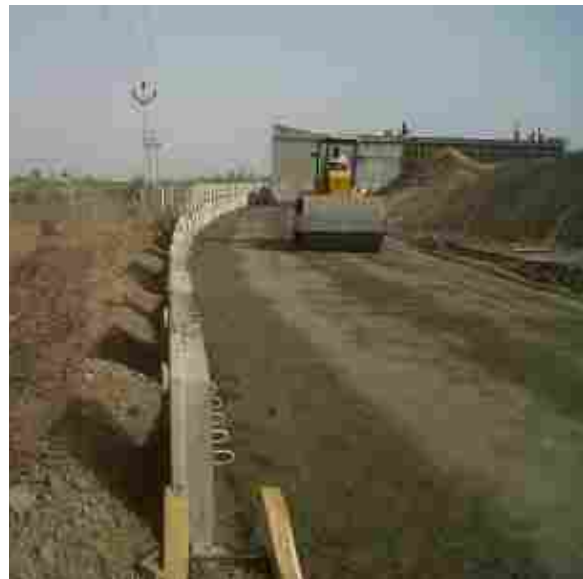
Photo 5. Spreading and Compacting the Reinforced Fill
