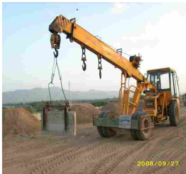
Photo 1. Lifting Arrangement for Panels
